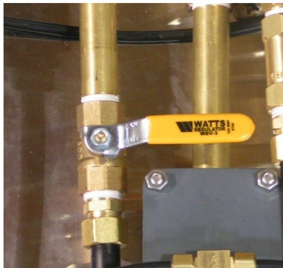
Figure 5-1. Filter Change Shut Off Valve shown CLOSED
