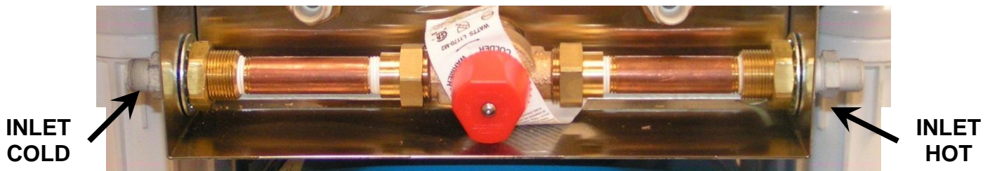
Figure 4-13. Blending Valve Assembly
