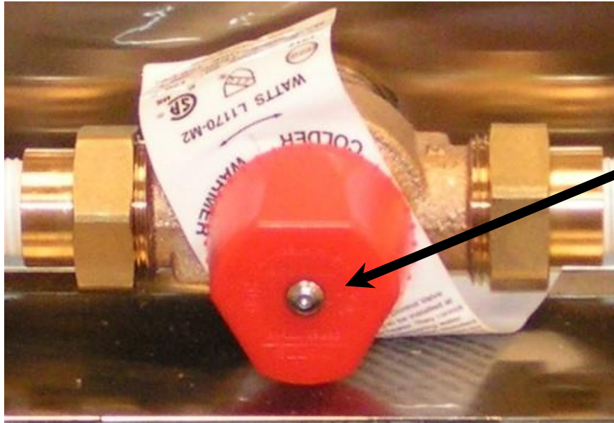
Figure 4-15. Blending Valve Locking Cap
