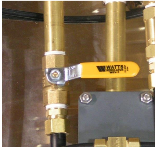
Figure 6-1. Filter Change Shut off Valve CLOSED
