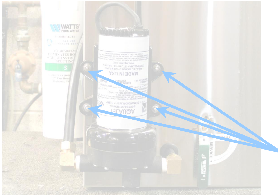
Figure 4-19. Low-Pressure Booster Pump Mounting Points
